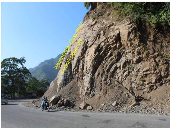
Figure 8. Slope profile section (B) showing the overall slope angle and the weathering grade.
