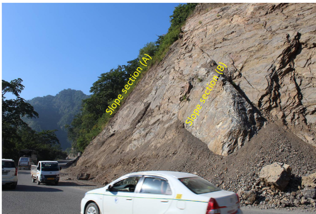
Figure 6. General overview of the investigated slope.
