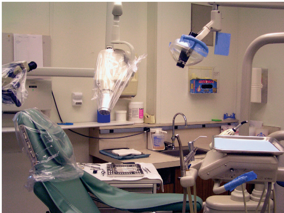
FIG. 6-14 Operatory plastic film barriers in place.
