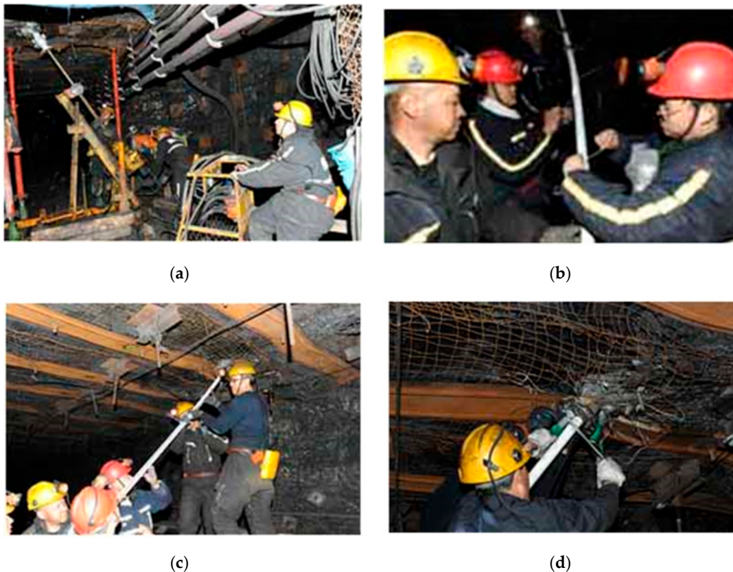
Figure 19. Process of embedding optical fiber in roof rock. (a) Drilling a borehole. (b) Fiber binding to the outer wall of PVC pipe. (c) Laying fiber through PVC pipe. (d) Grouting and sealing in borehole.
