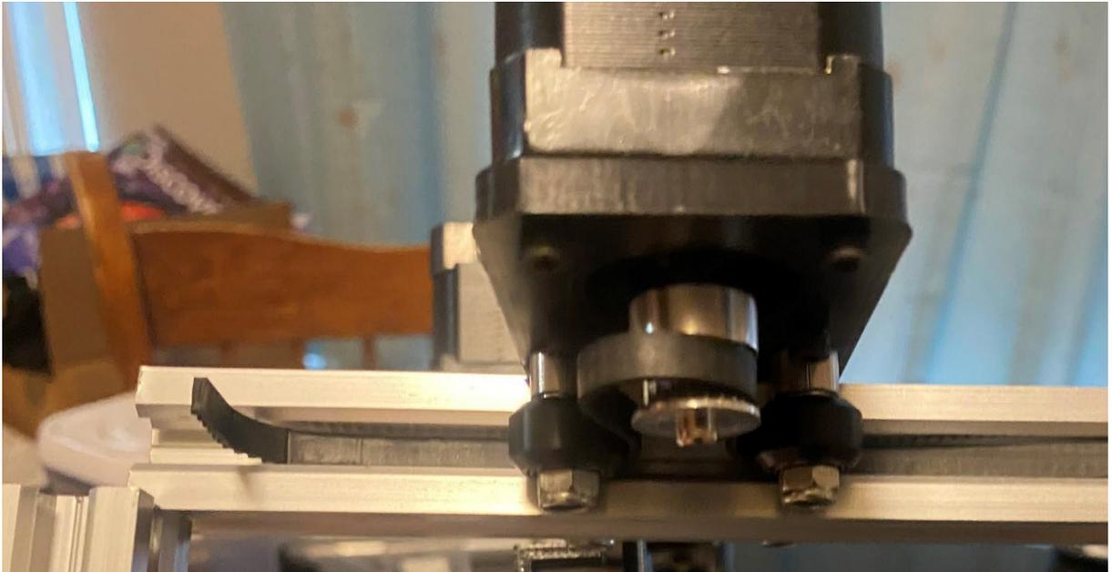
**Fig. 44.** Installing timing belt onto X-axis stepper motor.
