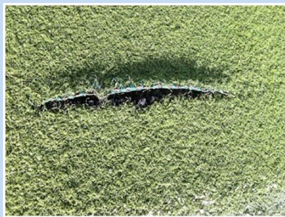
Figure 3. Seam damage.
