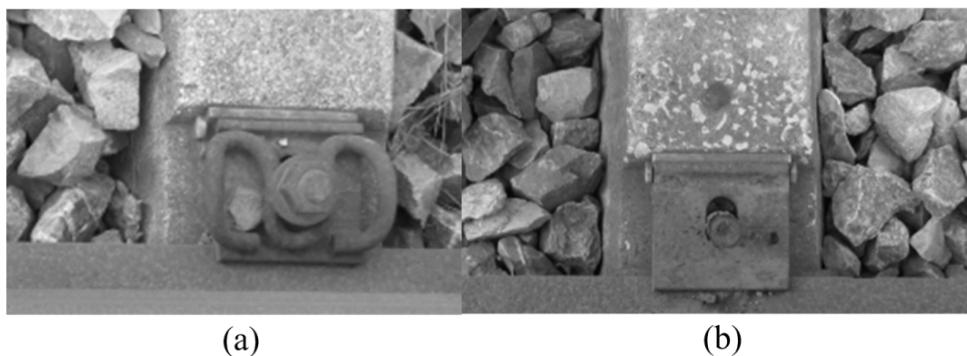
Figure 11. Matching and searching results from Figure 10 using the relevant DF pattern. (a) With a fastener; and (b) Without fastener.
