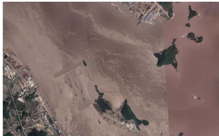
Figure 14. The water area at Zhoushan Xiushan Island (Google Earth 30^{\circ}08.00'' N and 122^{\circ}08.00'' E).
