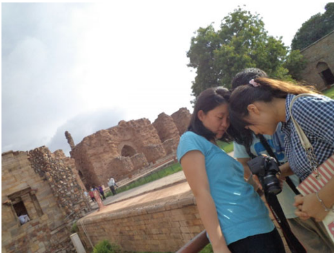
Fig. 1.3 Remnants of historic building with mud masonry in an Asian City
