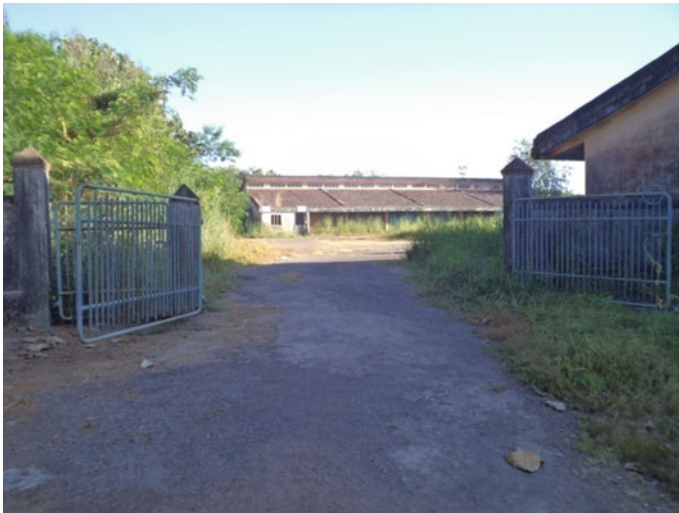
Fig. 1.20 Soiled walls and roofs in coastal area
