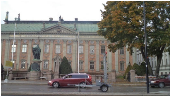
Fig. 1.7 Visible impact on statue and roofing due to acid rain
