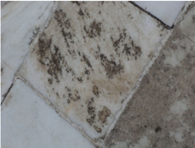
Fig. 1.18 Build up salts after attack of acidic air pollutants on marble used for flooring
