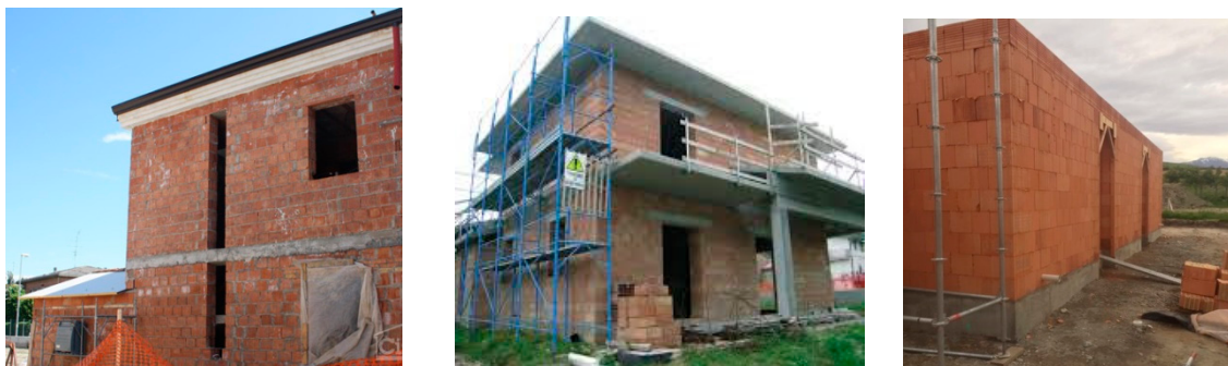
Figure 2. Example of residential block masonry buildings in Italy.
