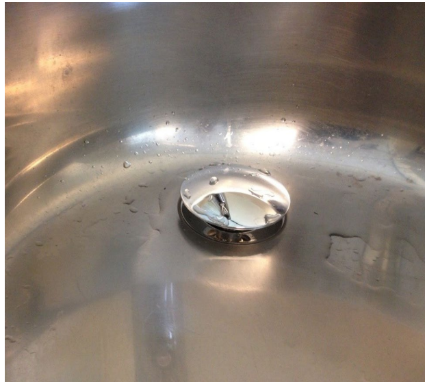
Figure 1. Drain plugs used in this study. Only sinks containing identical stainless steel drain plugs were considered for inclusion. The surface of these plugs contained no holes, and when screwed into the drain, completely covered the drain inlet.
