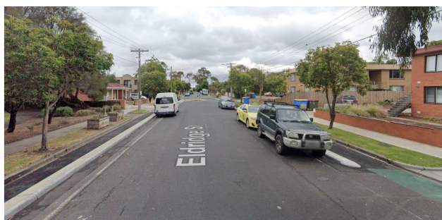
Figure 2. Google Street View screengrab of Eldridge Street Footscray, in Melbourne's inner west, showing recent retrofit of cycling lanes onto an existing residential street to include 300 mm physical barrier curb separation with 800 mm cycle path.
