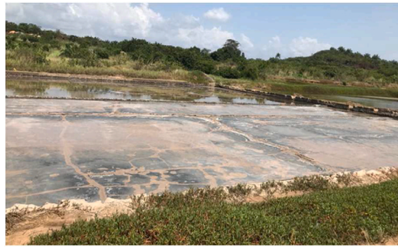
Fig. 3b. Concrete crystallization pans in KEEA, i.e., Elmina site, Dec 2022.
