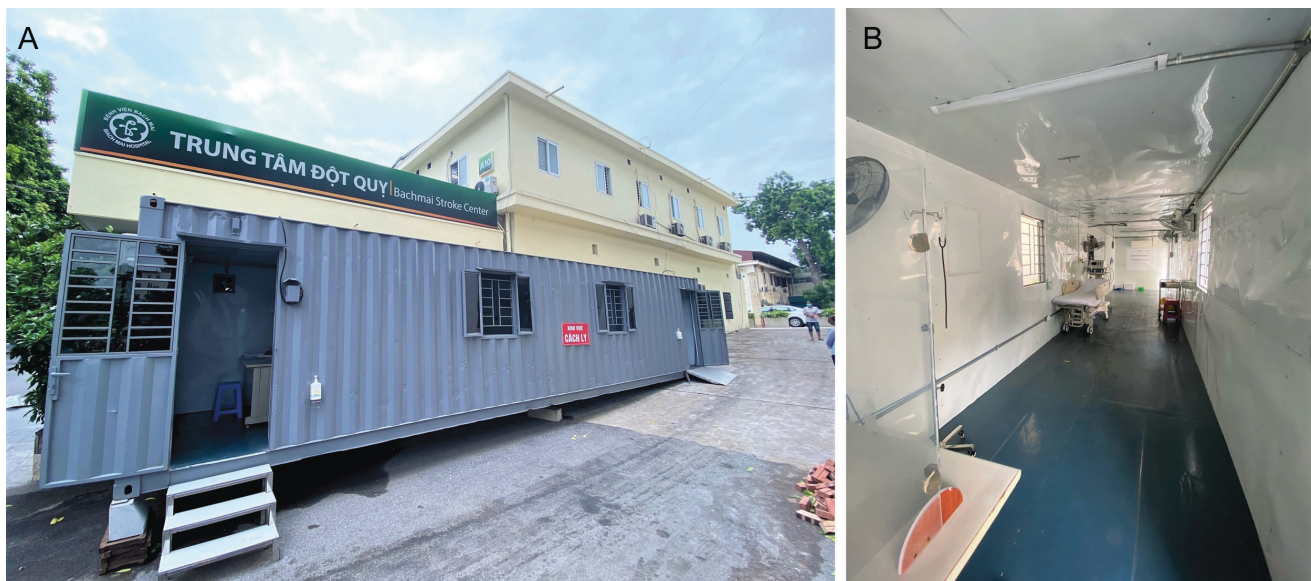
Figure 2. Shipping-container Stroke Isolation Unit at Bach Mai Hospital. Panel A. Front view. Panel B. Inside view.
