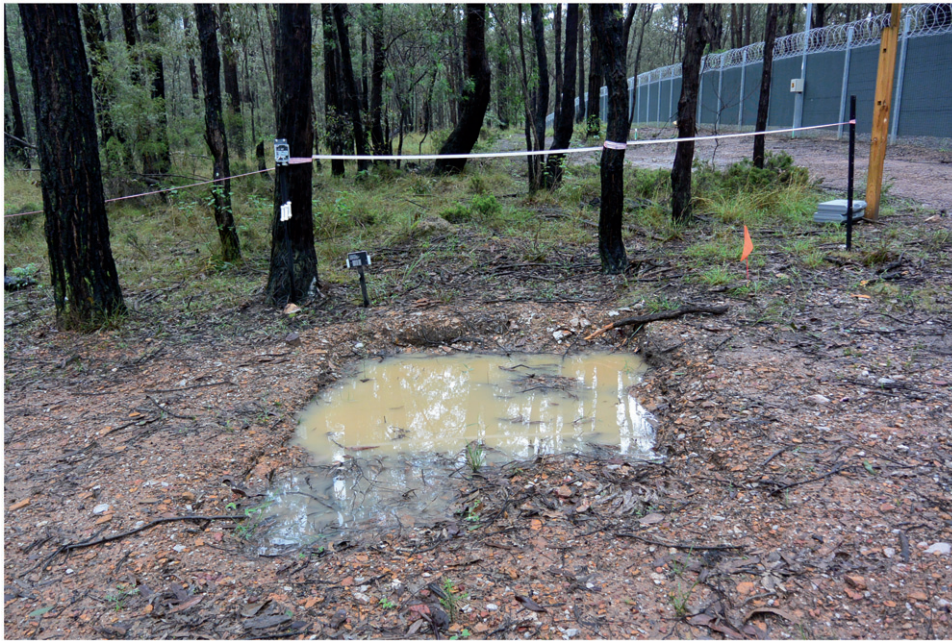
Figure 8. GR5 looking west showing obvious pooling of water, March 2017.
