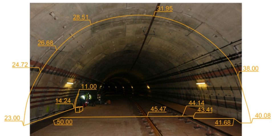
Figure 66. Monitored tunnel section [150].
