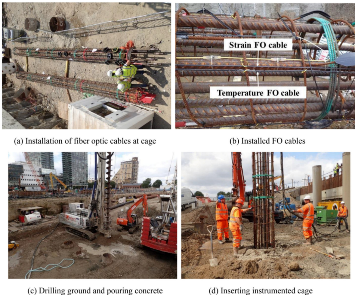
Figure 50. Installation of the DOFS and the pile [7].
