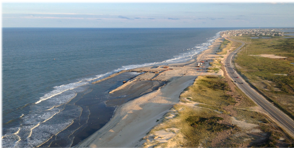
Fig. 2. Aerial view of the 2014 nourishment underway along the southern end of the Pea Island National Wildlife Refuge on the northern end of Hatteras Island. The populated Village of Rodanthe is set in the background.
