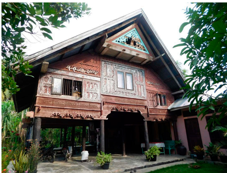
Figure 1. Traditional Acehnese house (stilt-style, with a single story) in Pidie Regency, Aceh, Indonesia. Lower right: semi-modern additional construction (combination of concrete and wood material; pink-wall), not part of the traditional house.
