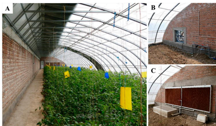
Figure 1. A solar greenhouse and the cooling devices used in the hot summer. (A), tomato plants and sticky card traps in a greenhouse; (B), cooling fan; (C), water curtain.
