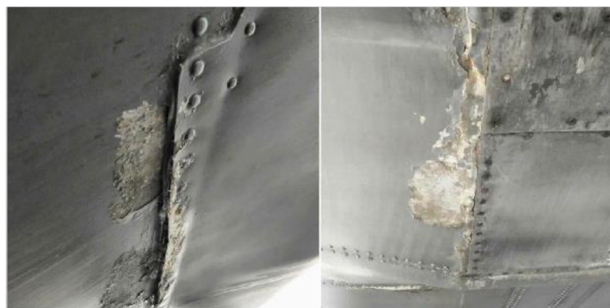
Figure 8. Corrosion at Lower Skin area.
