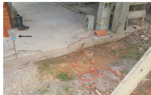
Fig. 1. Photograph from the injury scene revealing a protruding metal rod (arrow), now covered by a plastic water bottle after the incident for visibility.
