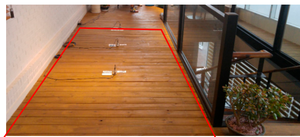
Figure 18. Cladding completion in Nambuk Church.
