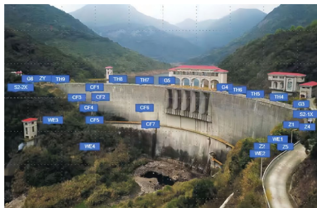
Fig. 2. Layout distribution map of dam monitoring points of XY Reservoir. (Author drawing).
