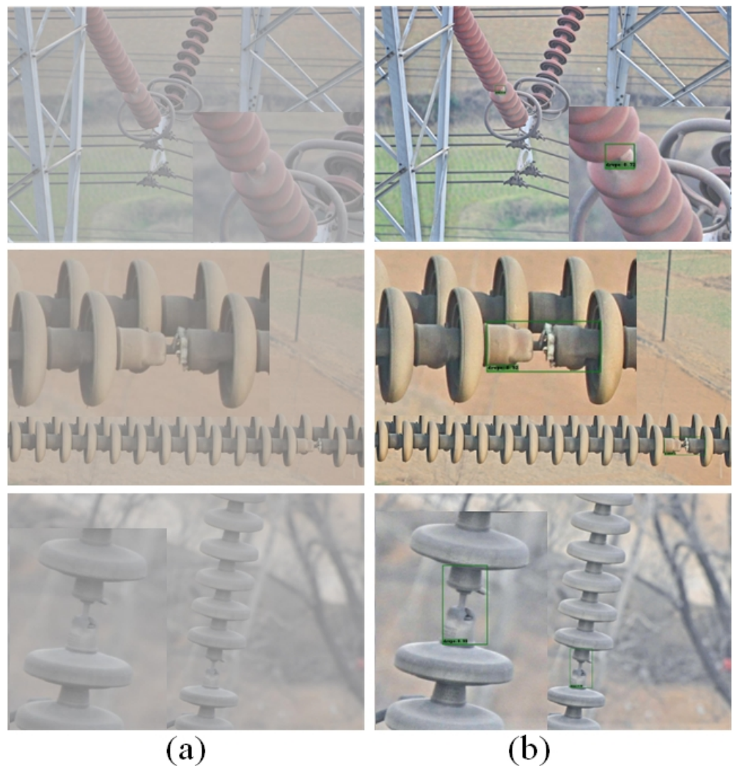
Figure 13. Visualization results of the FA-SSD and FA-SSD with defogging algorithm. (a) FA-SSD. (b) FA-SSD with defogging algorithm.
