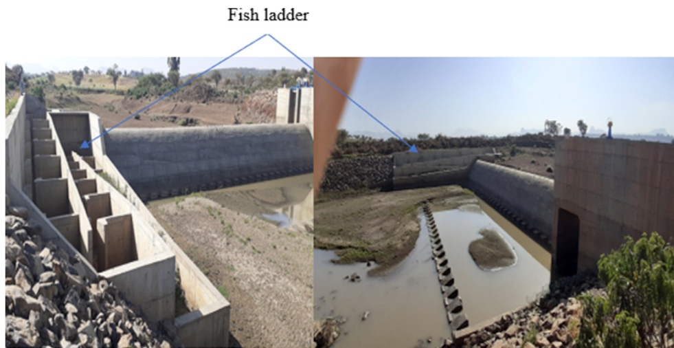
Figure 5. Fish ladder at Ribb Weir, on Ribb River.
