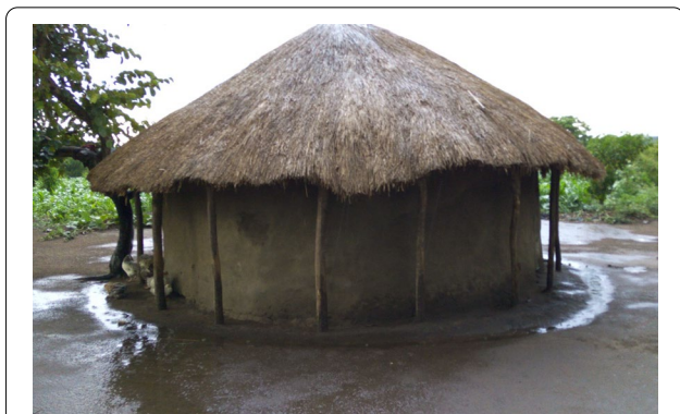
Fig. 2 Typical house used for aspiration of eaves. Of the 30 houses selected for eave aspiration, 24 had mud walls with grass-thatched, overhanging roofs and six were similar but with iron-sheet roofing material
