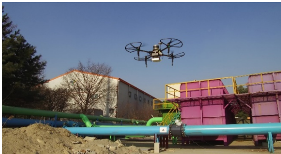
Figure 5. UAV on-site for the partial PCD acquisition using Velodyne Puck LITE.
