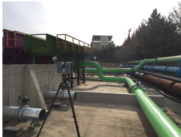
Figure 2. Pre-processed PCD acquisition using a Trimble X5 on-site.
