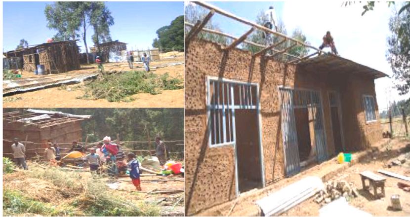
Fig. 6. Demolishing operation in Burayu city.
