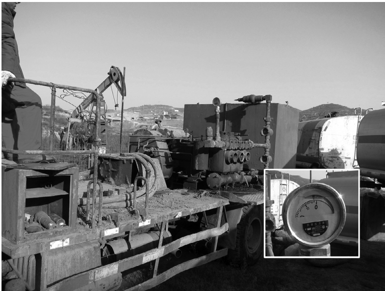
Fig. 2. On-site media injection and pressure control.
