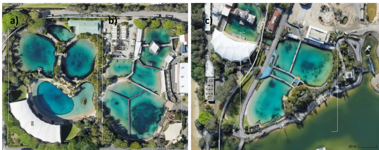
Fig. 1 Aerial view [37] of the three pool systems. a Dolphin Beach, b Dolphin Bay, c Endeavour) at Sea World where sampled dolphins were kept in. Even when partition gates between 'subpools' were closed, water flow between 'subpools' still was still retained. The image was obtained from Google Maps [37]
