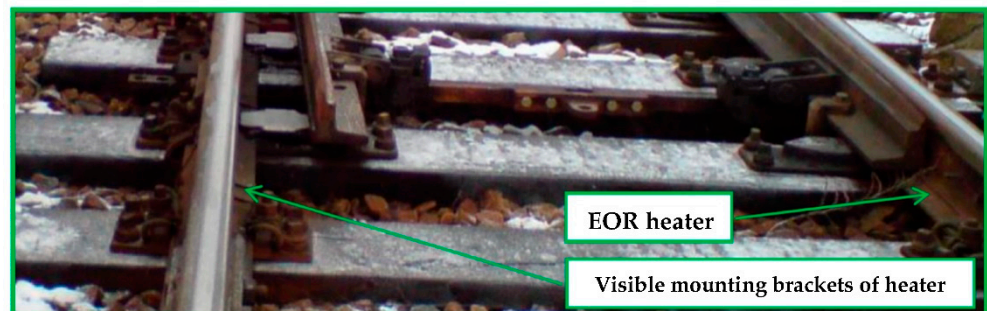
Figure 2. Enlarged area of the photo showing a fragment of the turnout track layout (source: authors).
