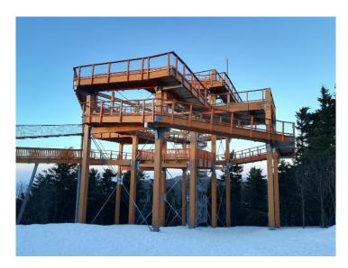
**Figure 1.** Example of a timber structure with bolted connections.
