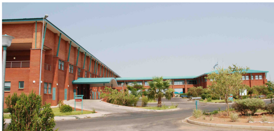
Fig. 2 Mahalapye District Hospital (Photo permission from Dr. Richard Brown via email on 24 October 2018)
