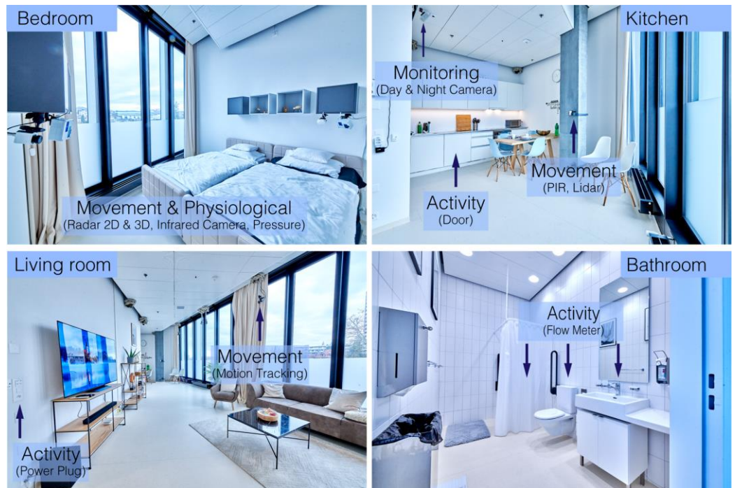
Figure 2. The instrumented apartment (NeuroTec loft): The installed sensors and their functions are indicated by blue shading.
