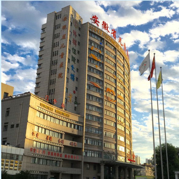
Anhui Provincial Children's Hospital: On the fast track to development
