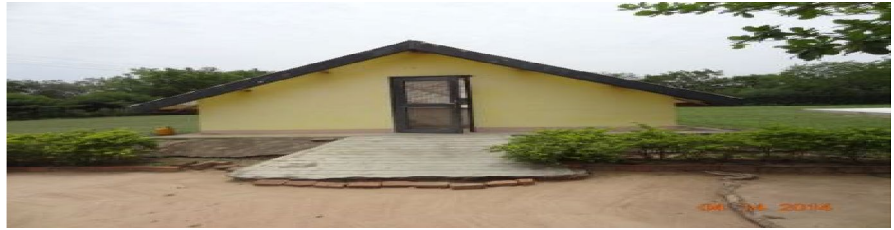
FIGURE 1 Pictorial representation of the tent-like concrete solar dryer (CSD)
