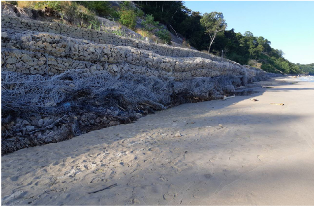
Fig. 2. Photo of coastal protecting structure (gabions in Svetlogorsk).
