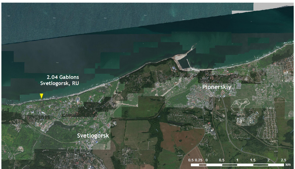
Fig. 1. General location of coastal protecting structures (gabions in Svetlogorsk) on the satellite image (Maps Data: Scanex Ltd., Image 2019 DigitalGlobe, Inc. CNES 2013, shooting year: 2019).
