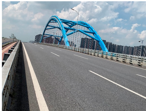
Figure 17. Current situation of the case bridge.
