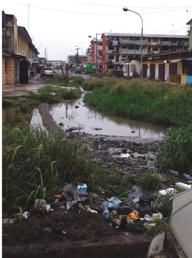
Figure 4. “This is another road. When it was initially built, it had distinct pedestrian way and motorist way but today, the road has been overtaken by weeds, all sorts of garbage and trash, and flood, smelling (stink), full of mosquitoes and flies. It is very closer to people’s houses (residence) such that even when you sleep the mosquitoes will not let you sleep well. This affects one’s motivation (for you) to get up in the morning and be healthy and to take one’s walk. One feels very weak because whenever you do not sleep well, you cannot get up healthy for activities, which is another challenge. Big one indeed.” Lady Susan (barrier).
