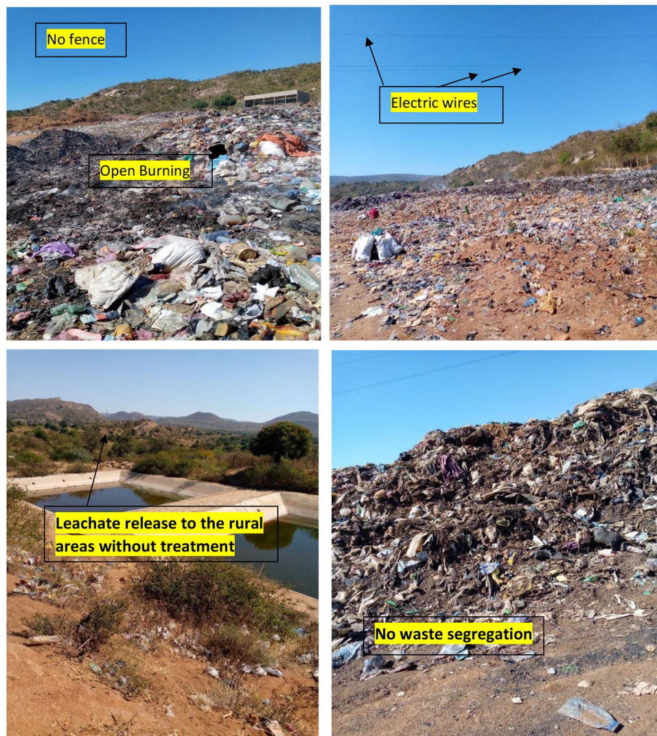
Figure A1. Harar city, Kile dumpsite, problematic and unscientific waste disposal site.
