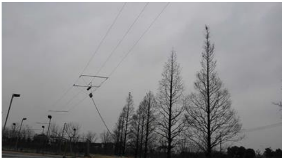
Figure 8. Erection image of 75 m three-wire transmitting antenna. It is a linear polarized dipole with the feed point in the center.
