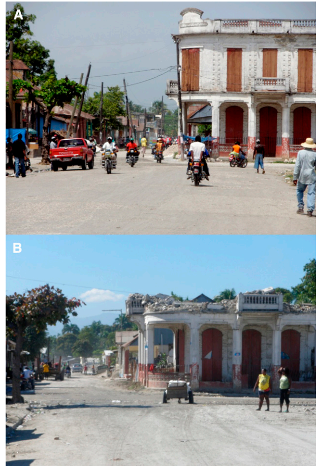
FIGURE 1. A and B demonstrate typical damage found throughout Leogane. (A) depicts one of the main thoroughfares of Leogane pre-earthquake. (B) depicts this same thoroughfare 1 year post-earthquake. Note the infrastructural damage, loss of electric poles, and general decrease in street activity.
