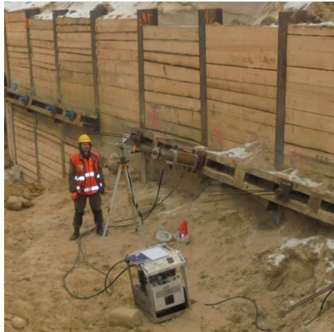
Figure 8. Details of excavation protection: load test of ground anchors.
