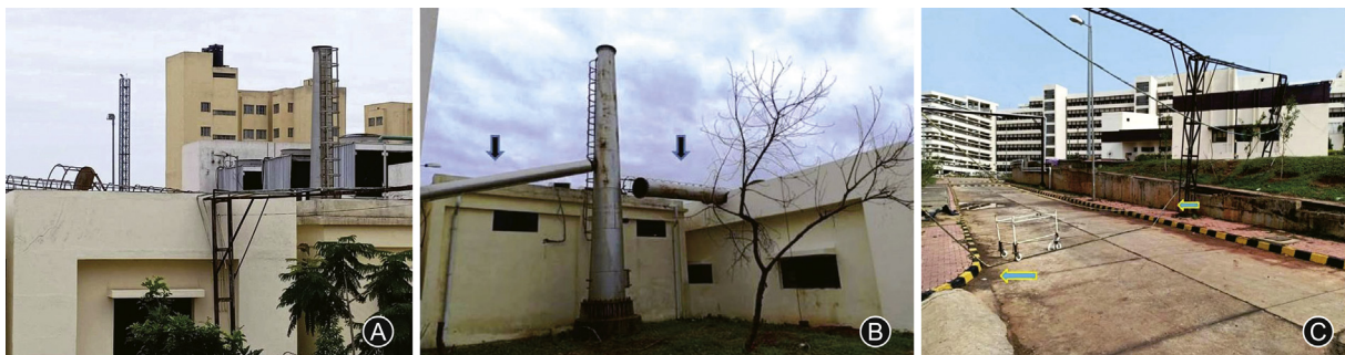
Fig. 4. (A) Broken chimney of boiling unit which fell on the medical gas pipeline system and central air conditioner coolant, causing damage to both; (B) Close view of the broken chimney parts (black arrow); (C) Disruption of medical gas pipelines (blue arrow).
