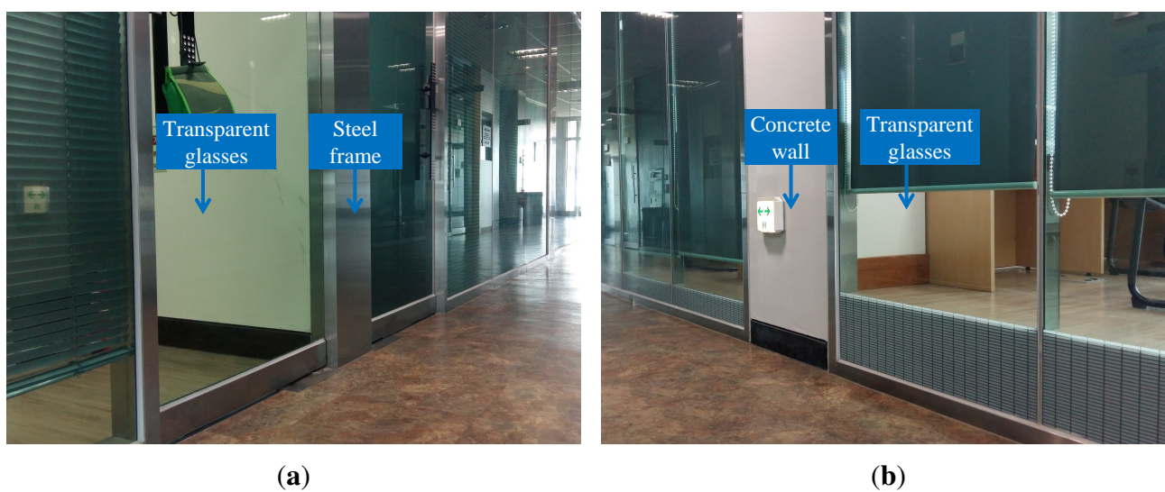
Figure 11. Snapshots of Dataset 3. Some parts of the wall are made of transparent glass. However, parts of the wall seen within the field of view consist of a steel frame or a concrete wall. (a) Steel frame with transparent glasses; (b) concrete wall with transparent glasses.
