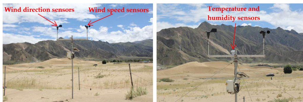
Figure 2. Wind-blown sand observation in the Shannan wide valley of the Sichuan–Tibet Railway.
