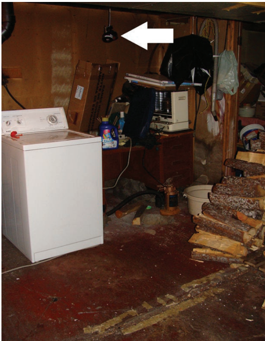
Figure 3: Electret hanging from the ceiling of the basement. The cracked floor is common in many basements of the surveyed houses.
