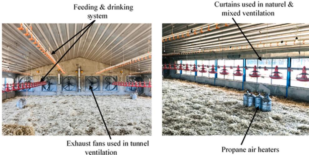
Fig. 2. Broilers house’s operational ventilation, feeding and heating system.
