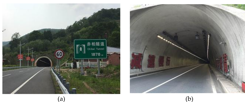
Figure 1. Chibai Tunnel, (a) Entrance to the tunnel; (b) LED luminaries installed in the tunnel.
