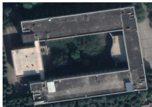
Figure 9. Optical scene of the roof.
