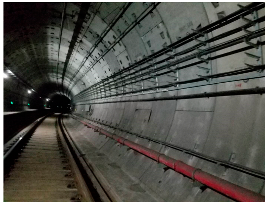
Figure 11. Practical working environment of the subway tunnel.
